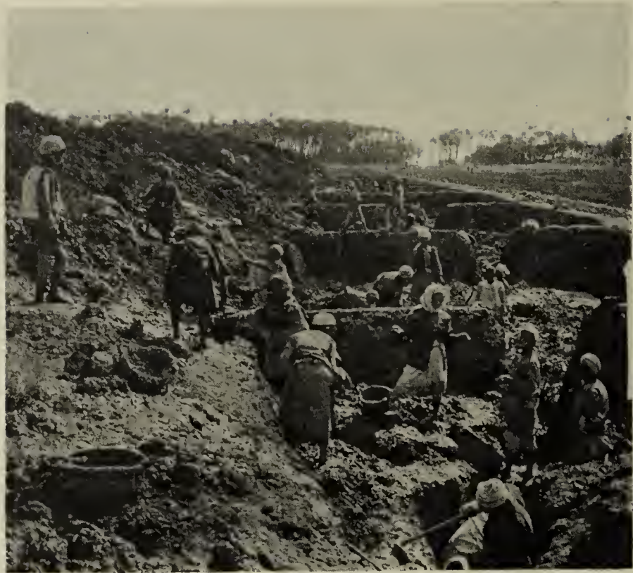
ABOUT 4 FT. DOWN WATER IS REACHED
